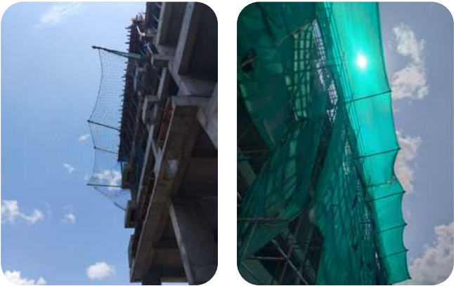
Figure 8. Safety nets installed for employee safety
