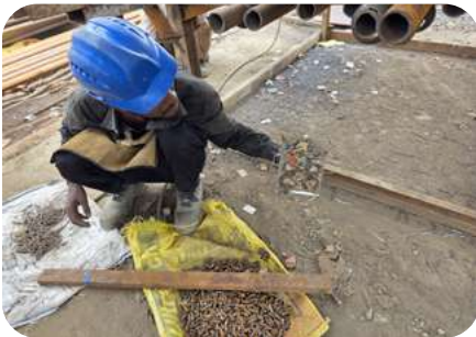
Figure 6. Nail catching with magnet at project site for worker safety
